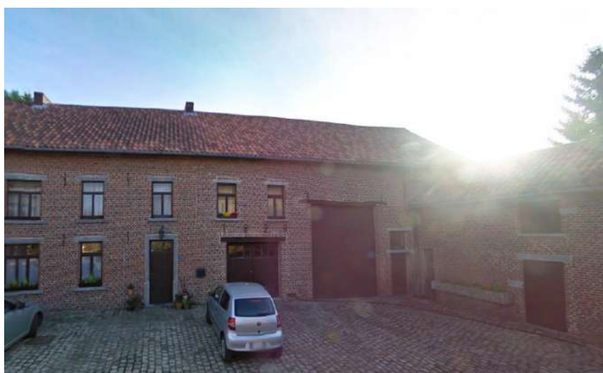
Figure 13 : Rue Trémouroux (Google Earth)
